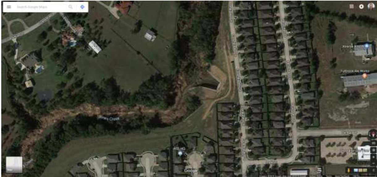
Rio Vista Street Storm Drain System Outfall into Jones Creek
